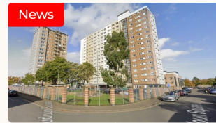
News Recladding of council high rises set to make further progress
