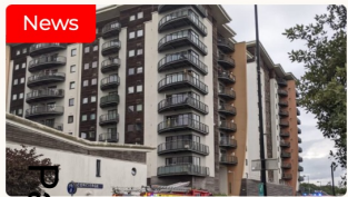
News Alarming fires in cladding hit Cardiff Bay building
