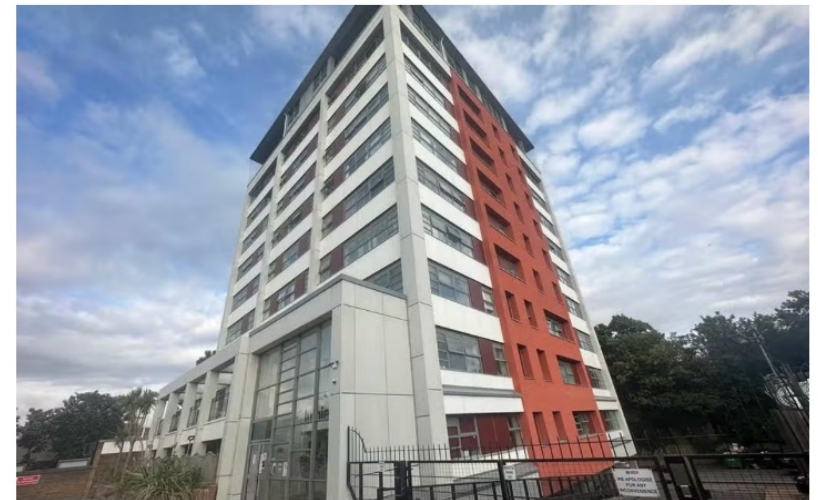
THE LUMIERE BUILDING IN FOREST GATE
